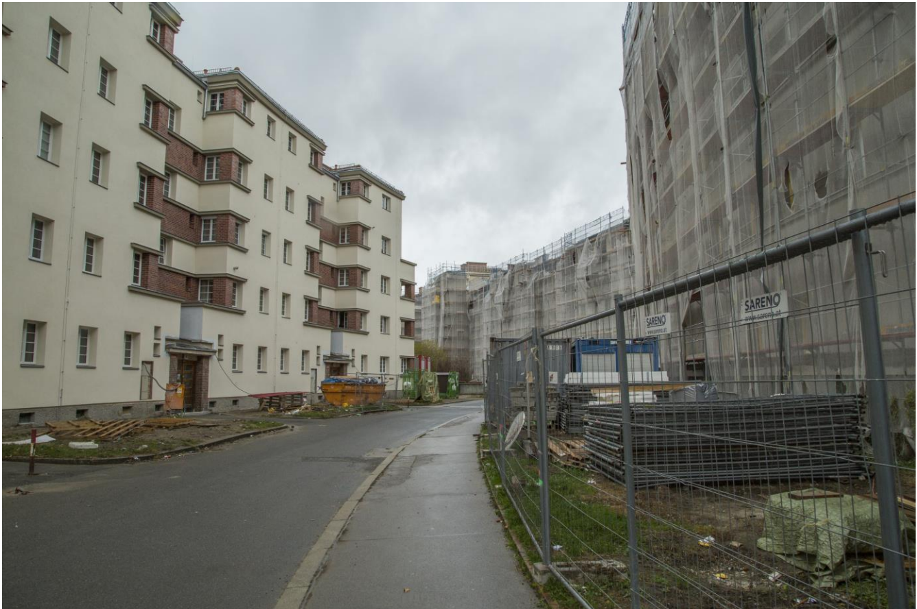
Refurbishment of the Goethehof (work in progress, 2015) ©J. Lodemann 2015
